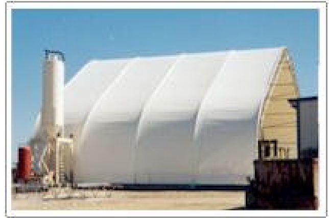
Figure 7 Sand blasting tent (industrial use)
