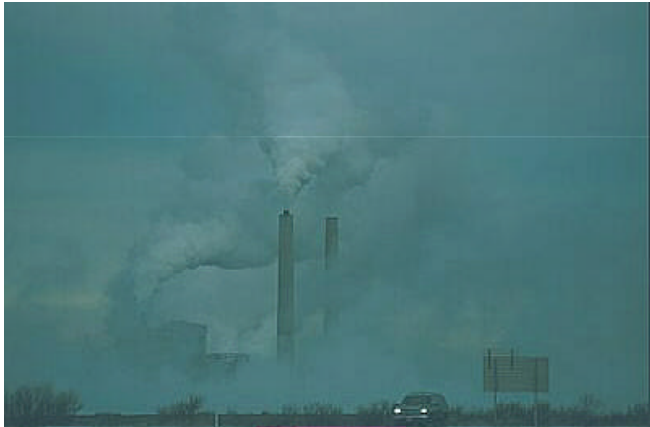
Figure 1. Coal-Fired Power Plant
