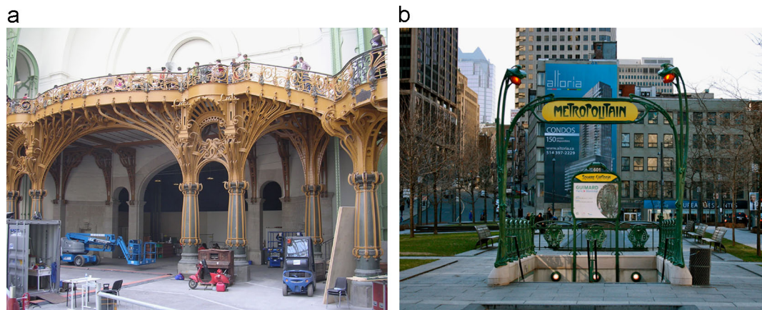
Figure 11 (a) Grand Palais in Paris built in 1900. (b) Entrance gate of Paris Metro designed by Hector Guimard in 1900.
