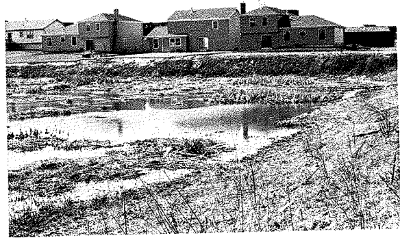
b. detention basins ( dry type ) Upper Photo: neatly graded, grass, fence, recreational opportunities Lower Photo: poorly graded, poor appearance, health hazard
