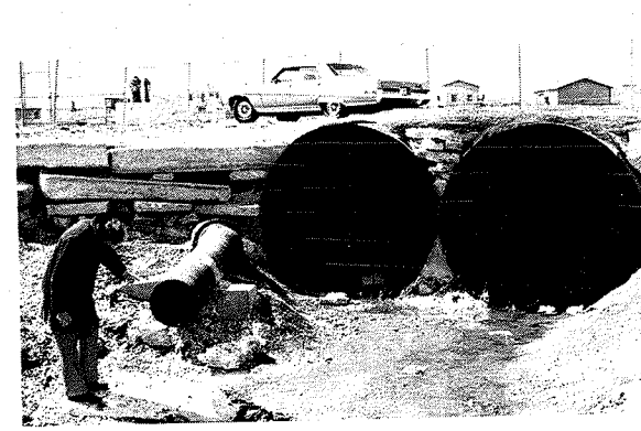
f. inlets to detention basins Upper Photo: safety features, neatly graded, debris grate, grass, long life Lower Photo: hazardous, unsightly, temporary life
