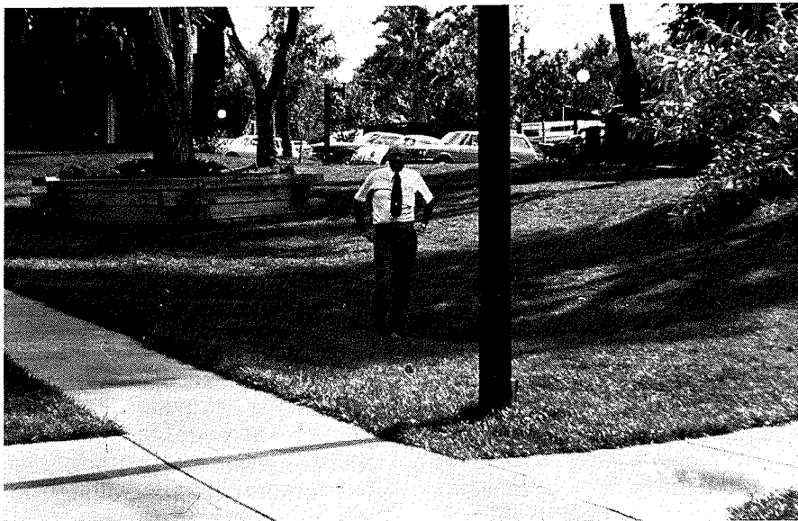
b. storm sewer inlets in grass areas restrict inflow rates
