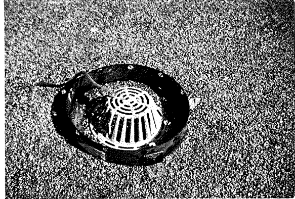
b. close-up of rainfall ponding ring and conductor head
