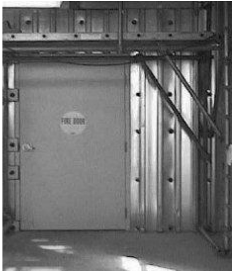
FIGURE 10.8: Heavy Steel Panel on Blast Side of Retrofitted Wall
