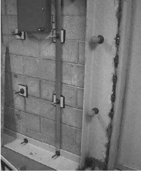
FIGURE 10.9: Through-Bolts on Inside Surface of Retrofitted Wall
