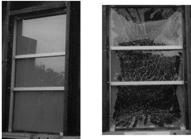
FIGURE 10.19: Window Retrofit Using Mullions and Film
