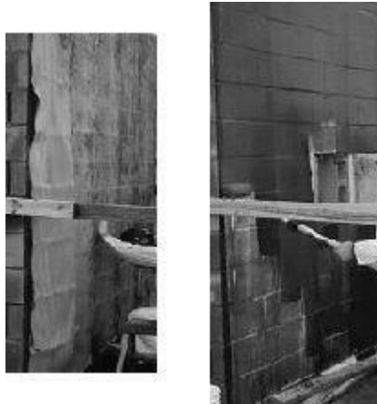
FIGURE 10.10: Kevlar® Wrap Retrofit to CMU Panel
