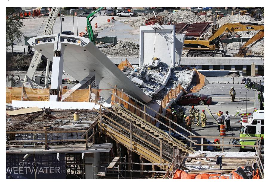
"On the day of the collapse, a construction crew was working on retensioning the post-tensioning rods within member 11, connecting the bridge canopy and the deck at the north end."
