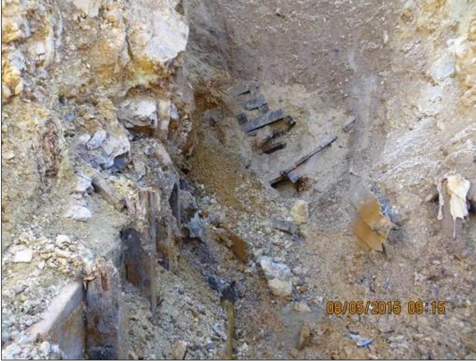
Figure 46.—Photograph taken at 9:15 a.m. August 5, 2015, showing the Gold King Mine Level 7 New Adit excavation uncovering mine timbers and lagging (photograph from EPA project files). Minor seepage is visible just to the left of the date stamp where a small puddle has formed. Note the soil in the upper end of the excavation above the timber lagging.
