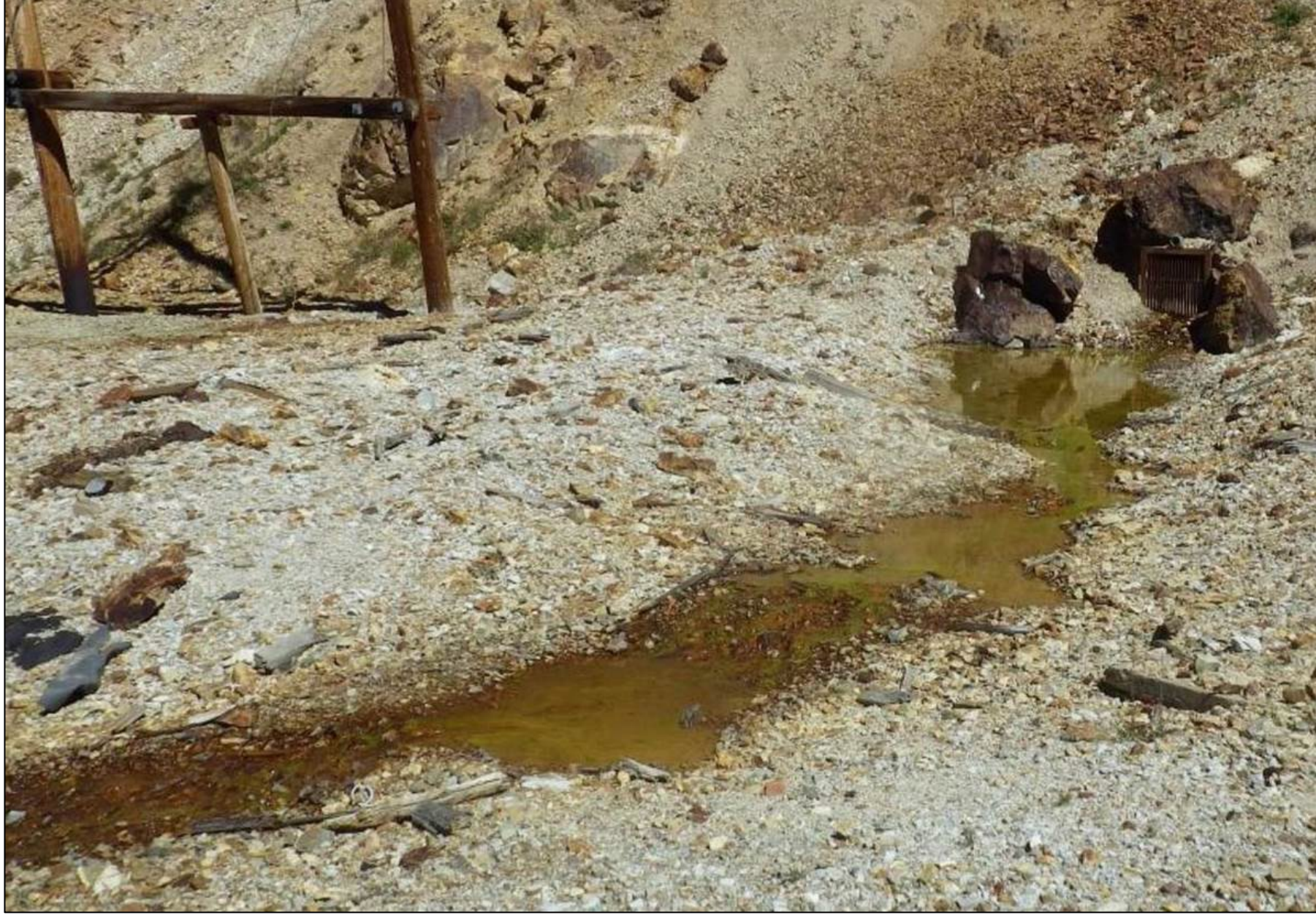
Figure 31.—Gold King Mine Level 7 OLD Adit (upper right) showing a small amount of seepage flow on September 11, 2014. At the portal, the floor of the old adit is approximately 2 feet higher than the floor of the old adit portal (photograph from EPA project files).
