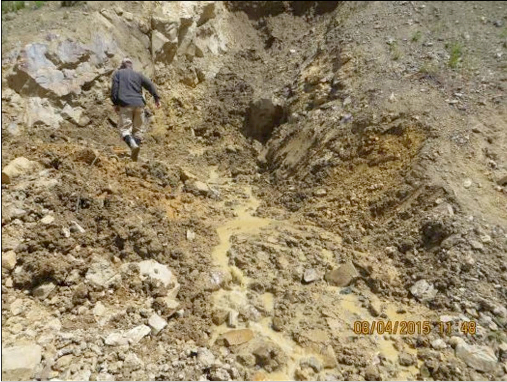
Figure 38.—Photograph showing seepage flow from the excavation at the Gold King Mine new portal at 11:48 a.m. on August 4, 2015. The flow is emerging approximately 5 to 6 feet above the floor of the adit (photograph from EPA project files).
