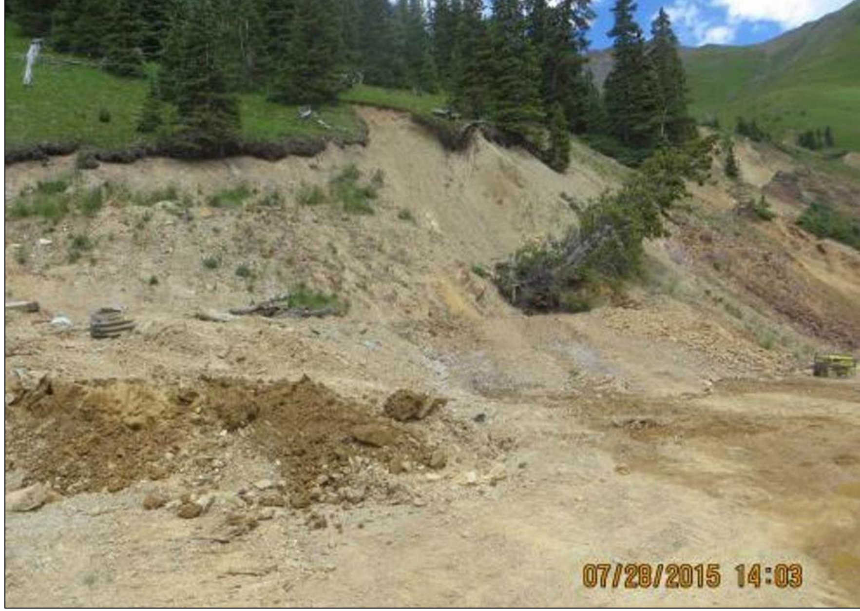
Figure 35.—Photograph showing the condition of the Gold King Mine Level 7 New Adit portal area on July 28, 2015. Note the soil and a tree that has slid downslope onto the portal area; at this time the seepage had been returned to the concrete trough, and the dump was drying out (photograph from EPA project files).
