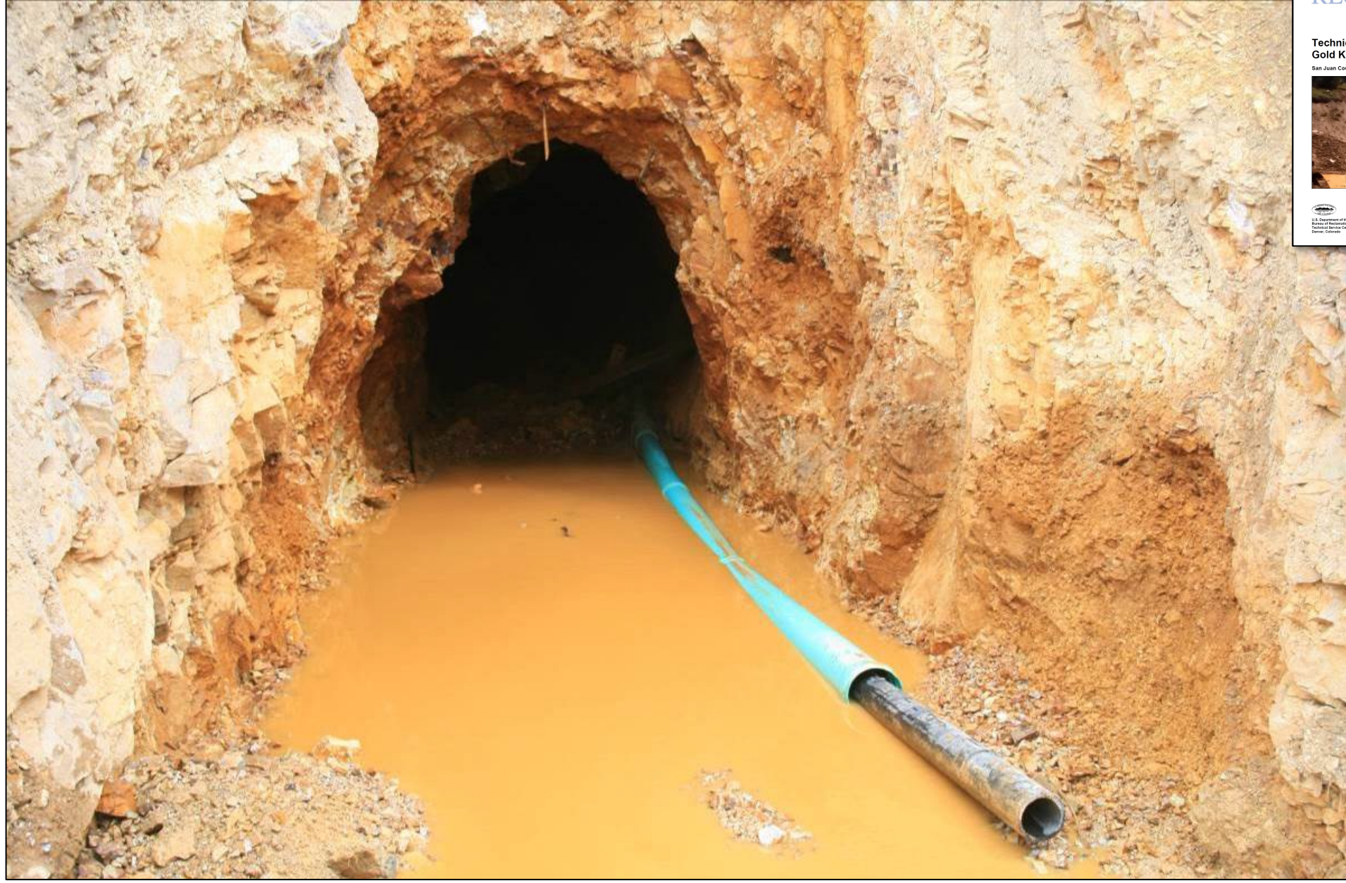
Figure 63.—Photograph showing the adit on August 16, 2015, with an 80-ft long (four 20-foot segments) turquoise-colored 24-inch outside-diameter drain pipe inserted into the adit opening. An 8-inch inside-diameter black HDPE pipe has been inserted into the 24-inch diameter pipe.
