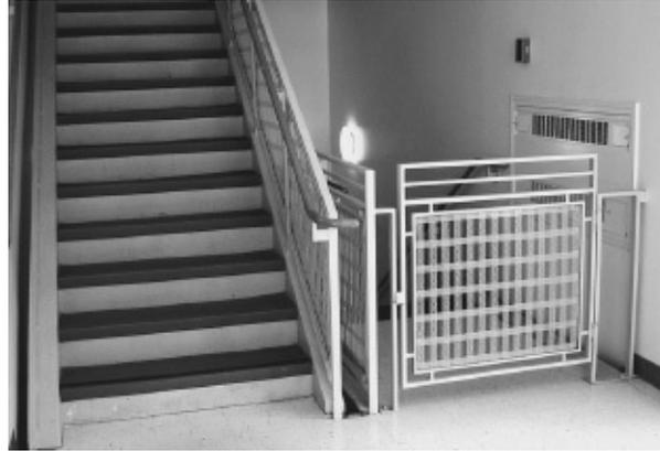
**FIGURE 4.7. A Lockout Forcing Function for Fire Exit.** The gate, placed at the ground floor of stairways, prevents people who might be rushing down the stairs to escape a fire from continuing into the basement areas, where they might get trapped.
