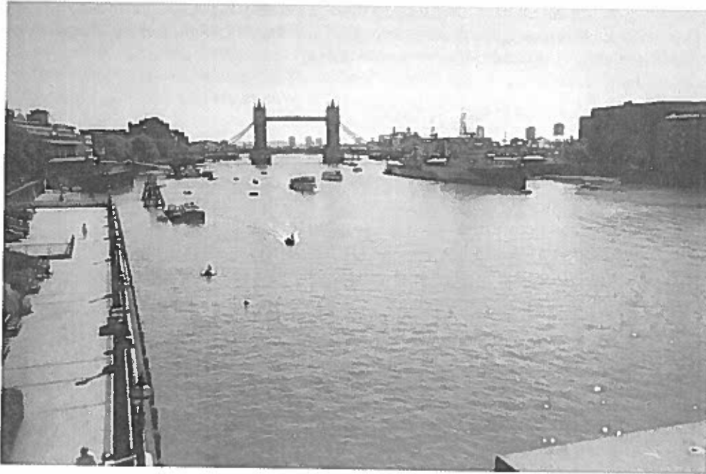
Figure 1.2 The London docks extend along 56 km of the 340-km Thames River. The river is the main water supply source for London. (Photo by R. A. Wurbs, May 1998)
