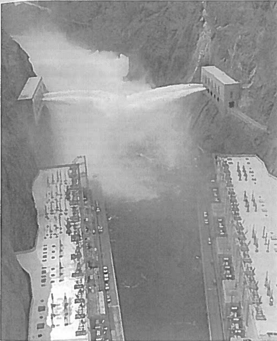
Figure 1.10 The USBR operates Hoover Dam to regulate the flow of the Colorado River to supply water for Las Vegas, Los Angeles, other cities, agricultural irrigators, and environmental instream flow needs; meet flow commitments to Mexico; generate hydroelectric power; and control floods. (Photo by W. P. James, June 1998)
