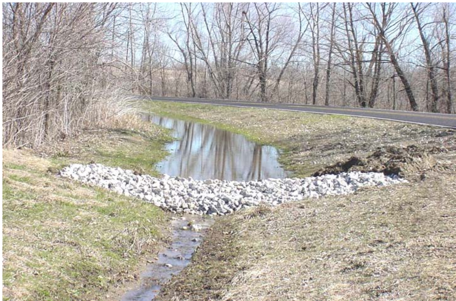
Figure 5.6 – Rock berm properly functioning to pool water.
