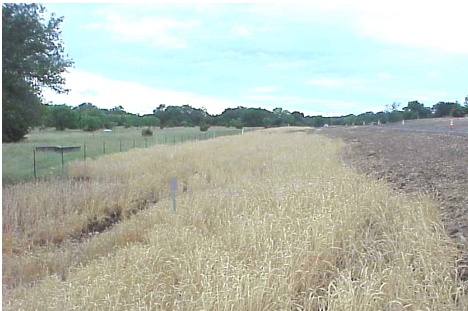
Figure 4.2 – Rye grass used to temporarily stabilize a slope.
