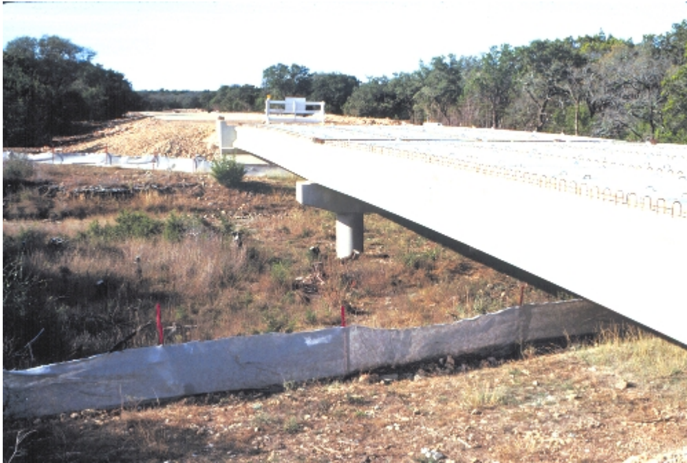
Figure 5.3 - Silt fence installed to protect a stream during bridge construction.
