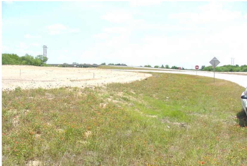
Figure 4.1 – Note extent of vegetation left in place.
