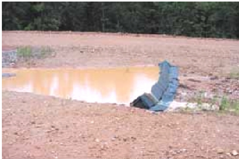
Figure 5.4 -Triangular filter dike
