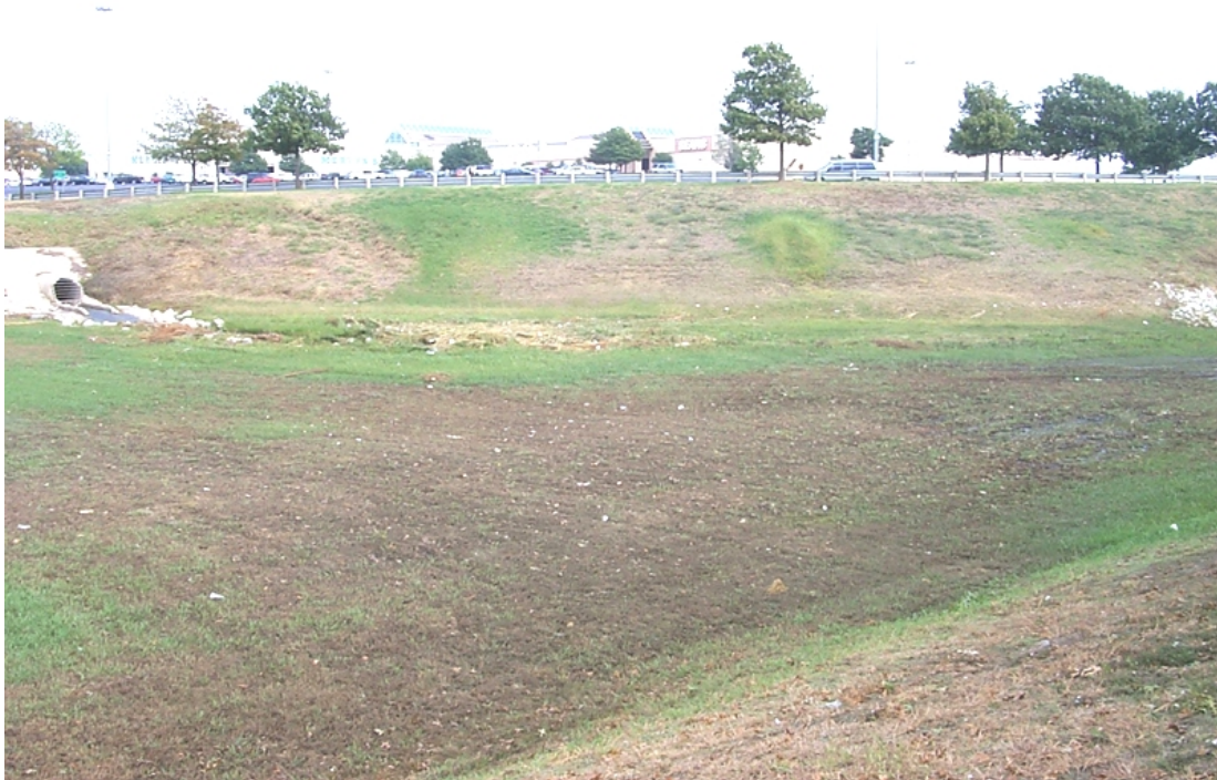
Figure 5.23 - Extended Detention Basin
