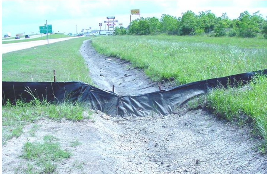
Figure 2.3 - Example of limiting disturbed area. Note the extent of vegetation left in place.
