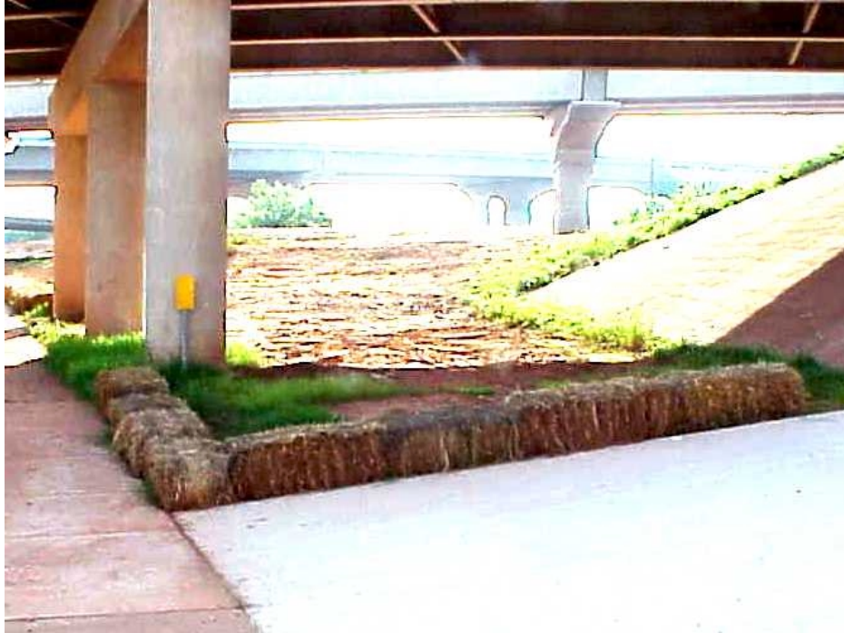
Figure 5.9 – Hay bales utilized to retain sediment onsite.
