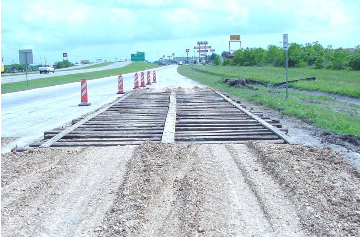
Figure 5.11 – Stabilized construction exit.
