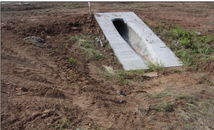
Figure 8-4. Pipe mitered to conform to fill slope.
