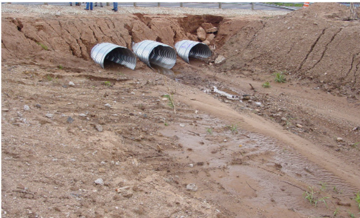
Figure 8-31. Temporary or Detour Culverts
