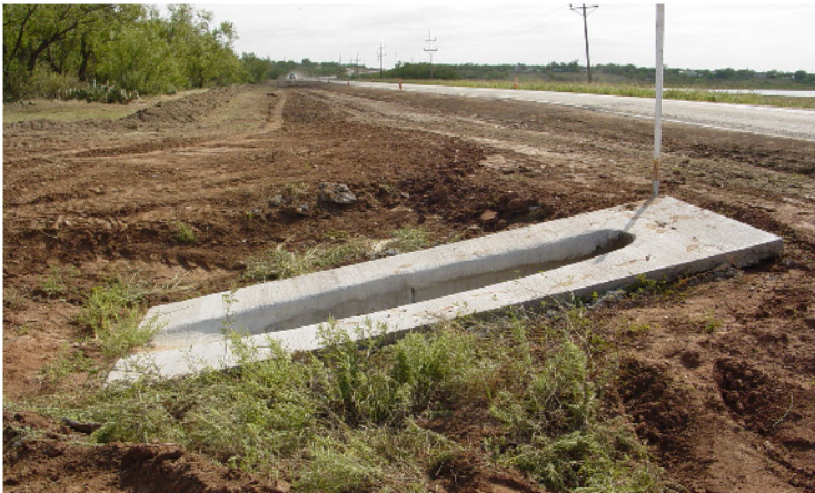
Figure 8-3. Pipe mitered to conform to fill slope.
