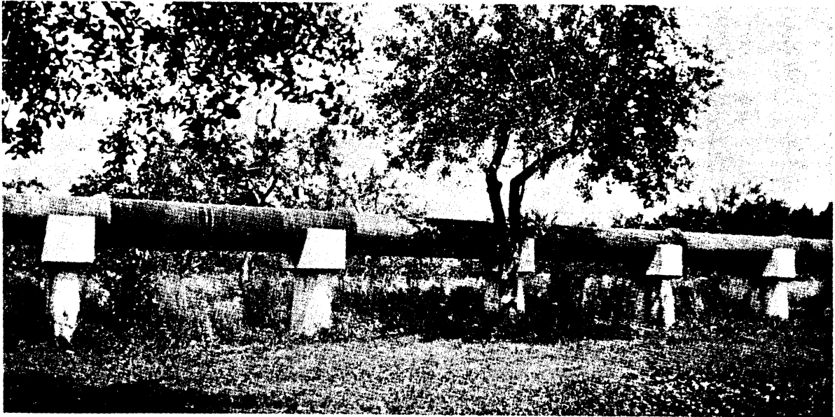
Figure 16-17 Sewer supported on piers.
