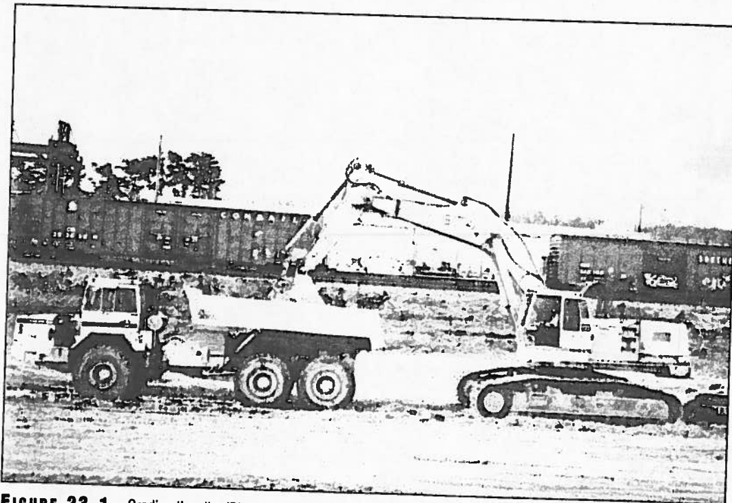
FIGURE 23.1 Grading the site. (Photo courtesy of Christer Carshult)
