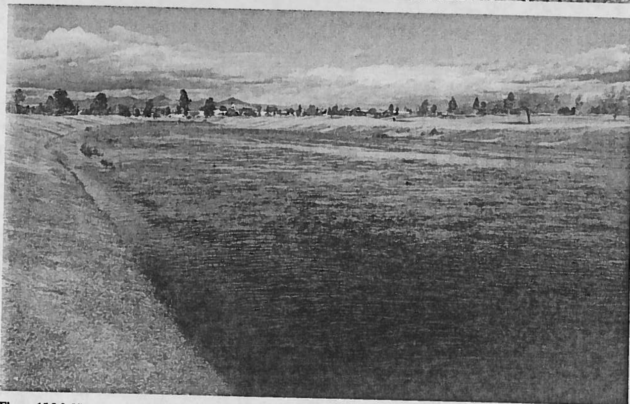
Figure 15.3.2 Views of Indian Bend Wash in Scottsdale, Arizona. The constructed channel is uniform and cross-sections are trapezoidal in shape (channel bottom is firm earth with seasonal growth of grasses and small brush) (Phillips and Ingersoll (1998)).
