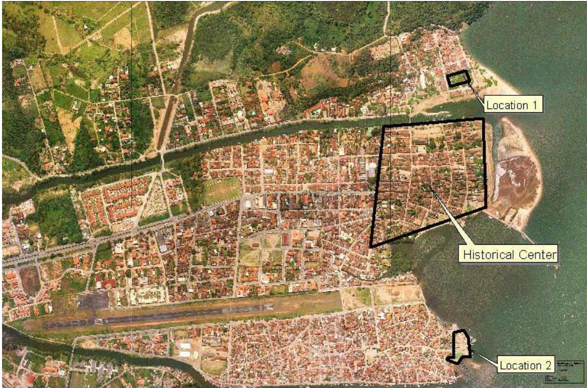
Figure 3.2 Aerial Photo of Paraty – Potential Locations of Treatment Plant 27 .
