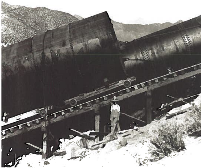
Where the aqueduct had to cross deep canyons, Mulholland employed inverted steel pipe siphons, the most impressive of which was in Jawbone Canyon, above . Construction required hauling huge pipe sections up steep slopes, left . Workers cover the conduit with cast-in-place concrete, below , in the Mojave Desert.
