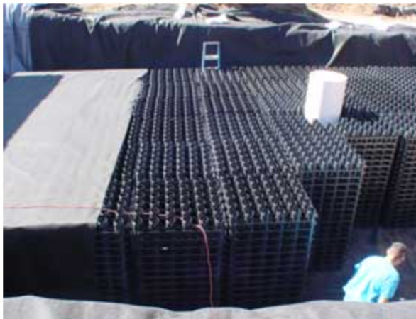
Rainstore 3 is perfect for water harvesting. two layers of geotextile fabric encase an impermeable liner. A maintenance/access port is shown.
