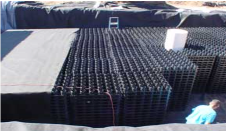
Rainstore 3 is perfect for water harvesting. two layers of geotextile fabric encase an impermeable liner. A maintenance/access port is shown.
