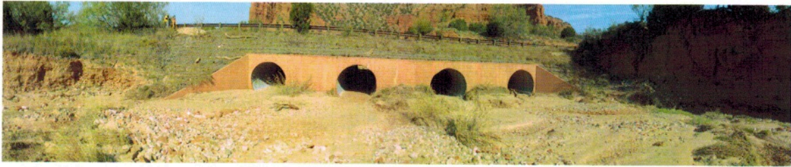
Figure 3: Multiple-barrel outlet structure
