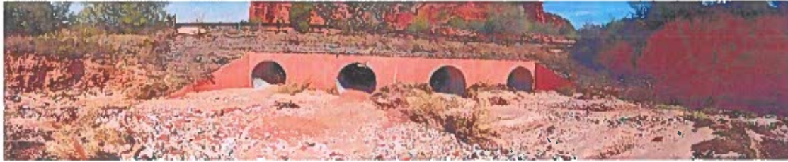
Figure 5: Multiple-barrel outlet structure
