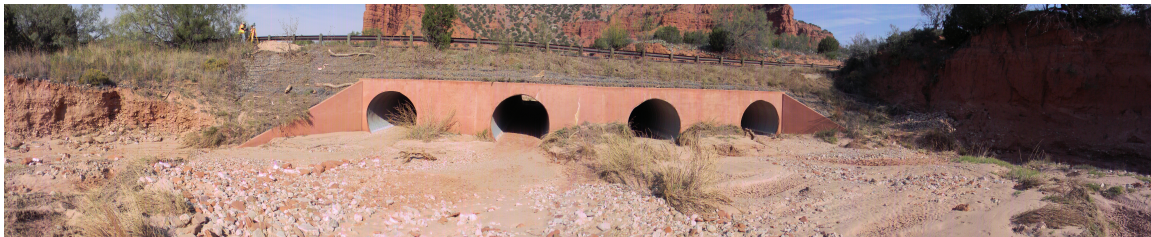
Figure 4: Multiple-barrel outlet structure
