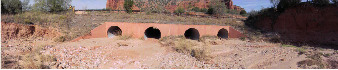
Figure 5: Multiple-barrel outlet structure
