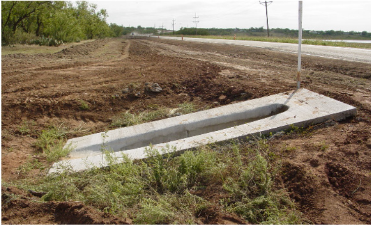
Figure 8-3. Pipe mitered to conform to fill slope.
