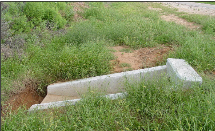
Figure 8-5. End section conforming to fill slope
