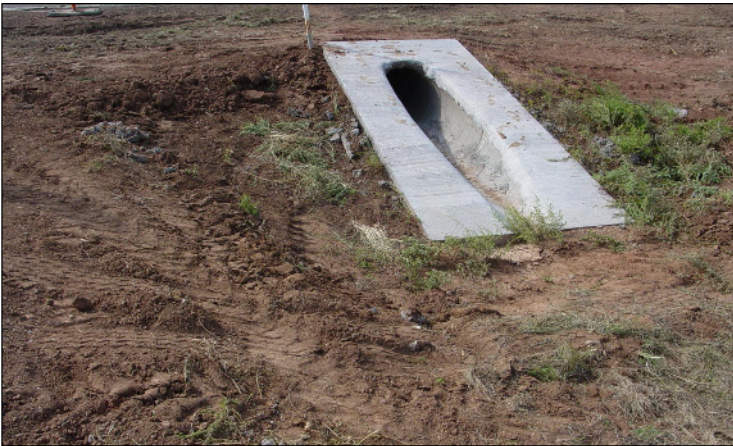
Figure 8-4. Pipe mitered to conform to fill slope.
