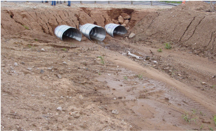
Figure 8-31. Temporary or Detour Culverts
