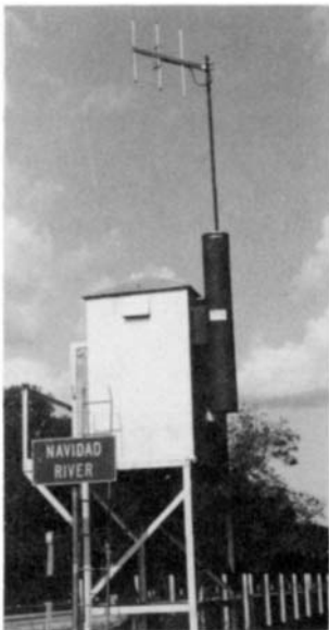
FIGURE 6.5.5 Self-reporting rain and water level gage on the Navidad River, Texas. (Courtesy of Sierra/Misco, Inc., 1986. Used with permission.)
