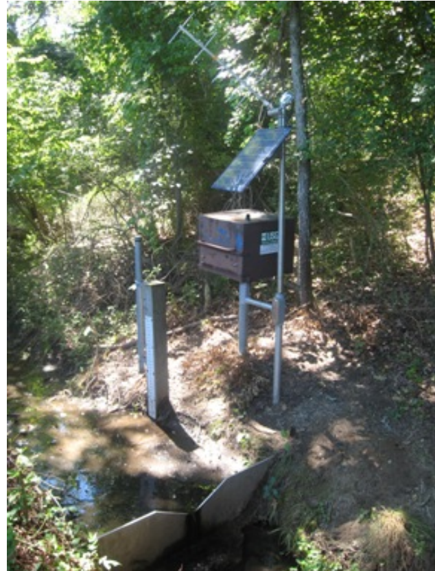
Figure 1. Photograph of a streamflow-gaging station showing a water-stage recorder, sharp-crested weir and crest-stage gage at U.S. Geological Survey station 01589238, Gwynns Falls Tributary at McDonogh, Maryland.
