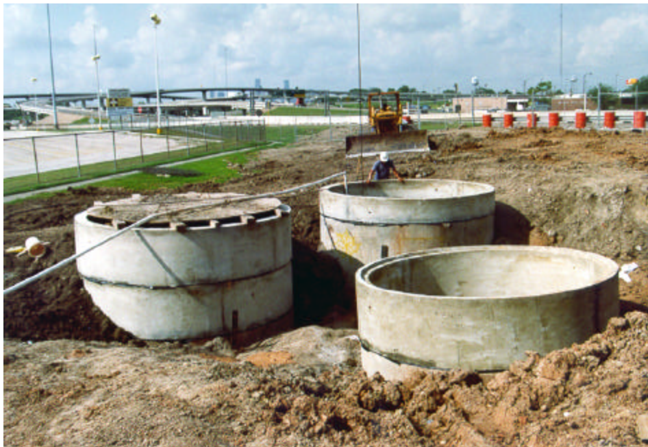
Figure 3-14. Circular caisson wet wells under construction.
