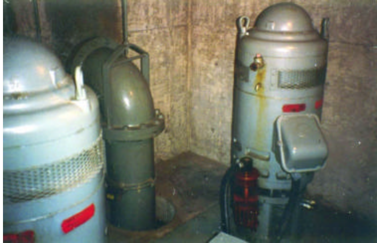
Figure 11-2. Typical electric motors for vertical pumps
