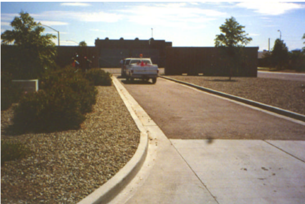
Figure 5-4. Driveway access to pump station in Arizona
