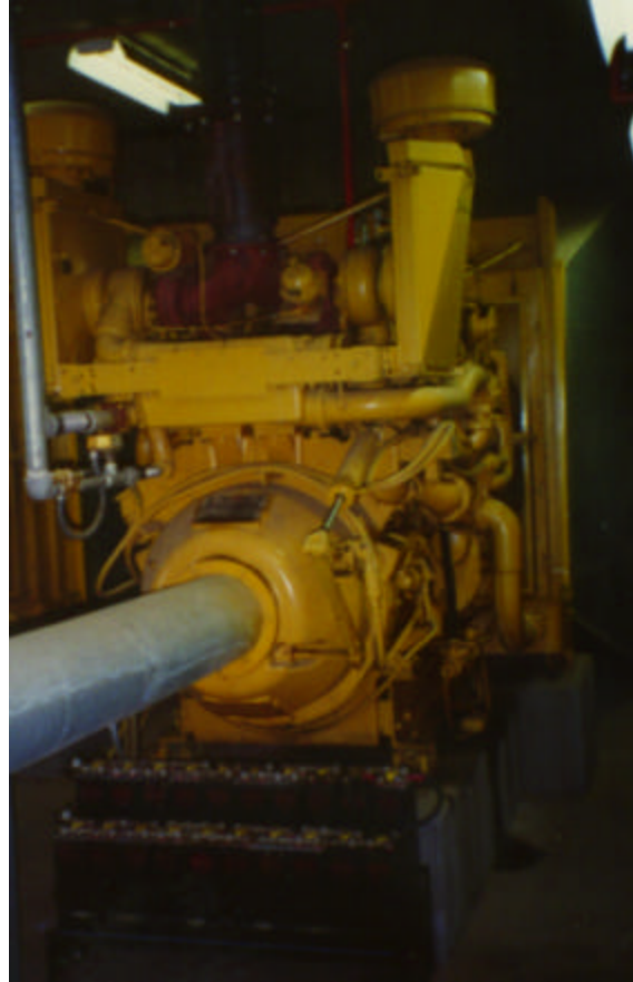
Figure 11-3. Engine drive
