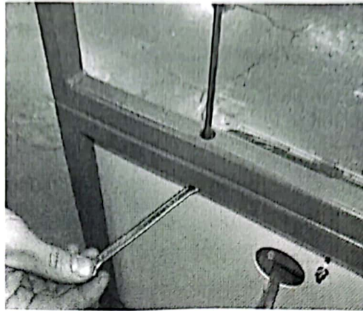
Figure 16 Fix the Instrument Rail to the Top of the Back Panel
