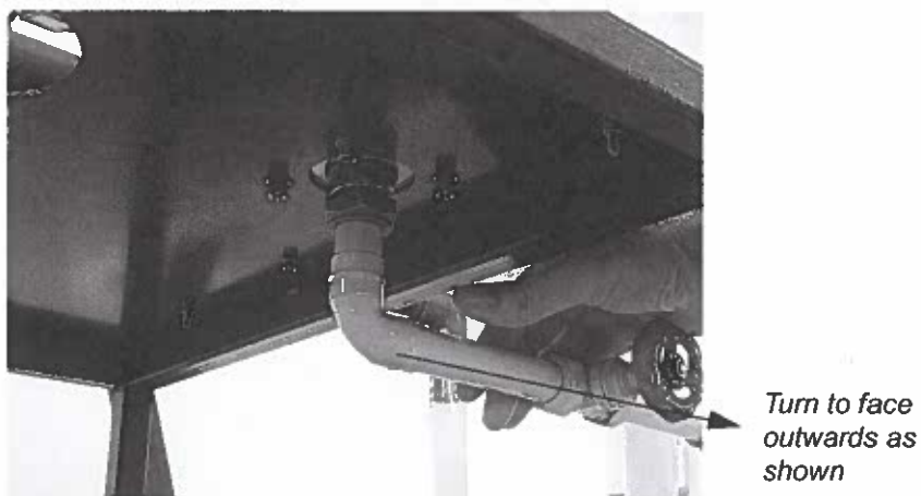
Figure 12 Rotate the Water Hammer Outlet Pipe to face Outwards as Shown
