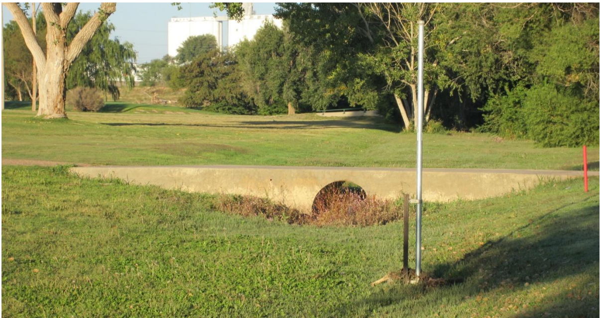
Figure #. View of the most upstream culvert and the upstream gage.
