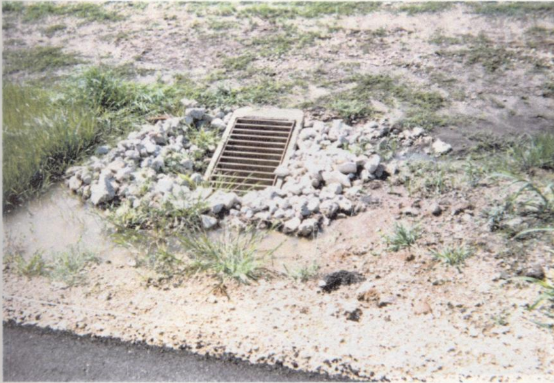
Figure 4: Rock Filter Dam TSC-4
