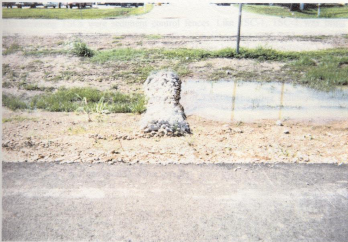
Figure 3: Rock Filter Dam TSC-3
