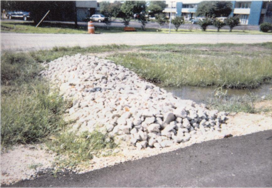
Figure 2: Rock Filter Dam TSC-1
