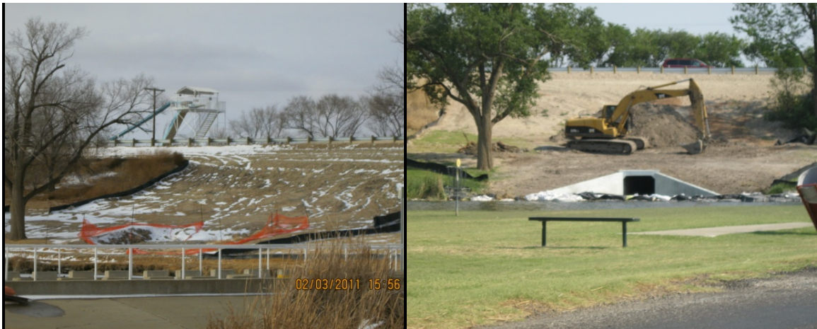
Figure 5. Marsha Sharp Freeway Discharge Location
