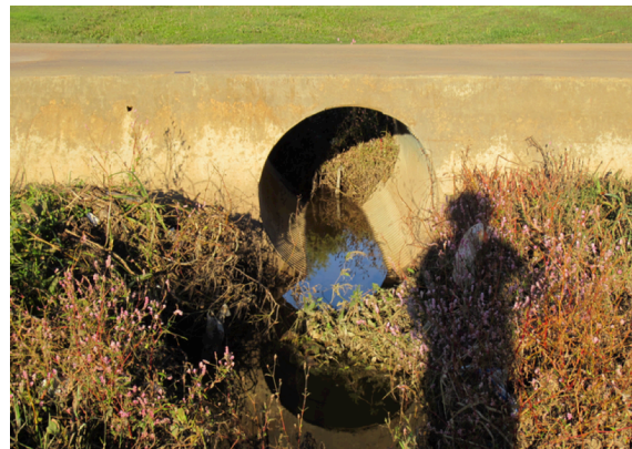
Figure 9: Downstream of Bridge Crossing C
