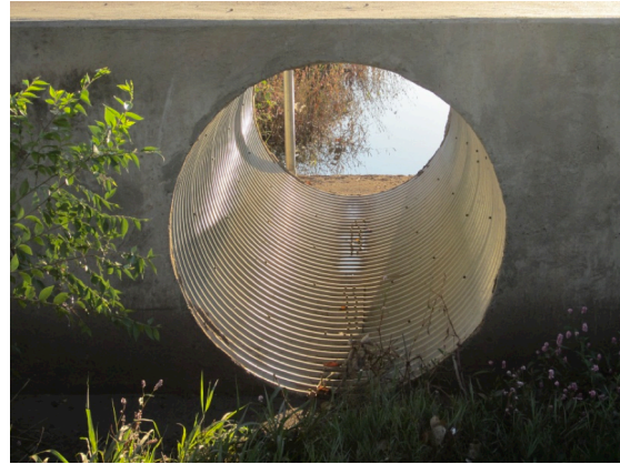
Figure 7: 48in Diameter Corrugated Metal Culvert
