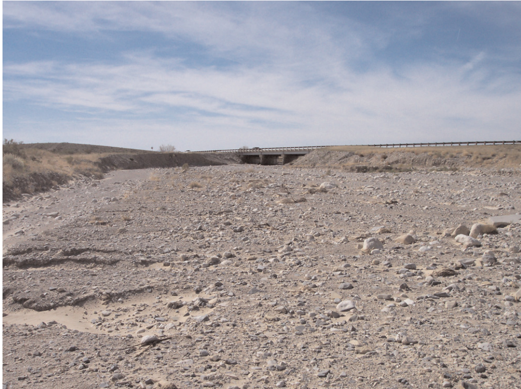
Figure 2.4. Streambed material (view of streambed looking downstream toward bridge).
