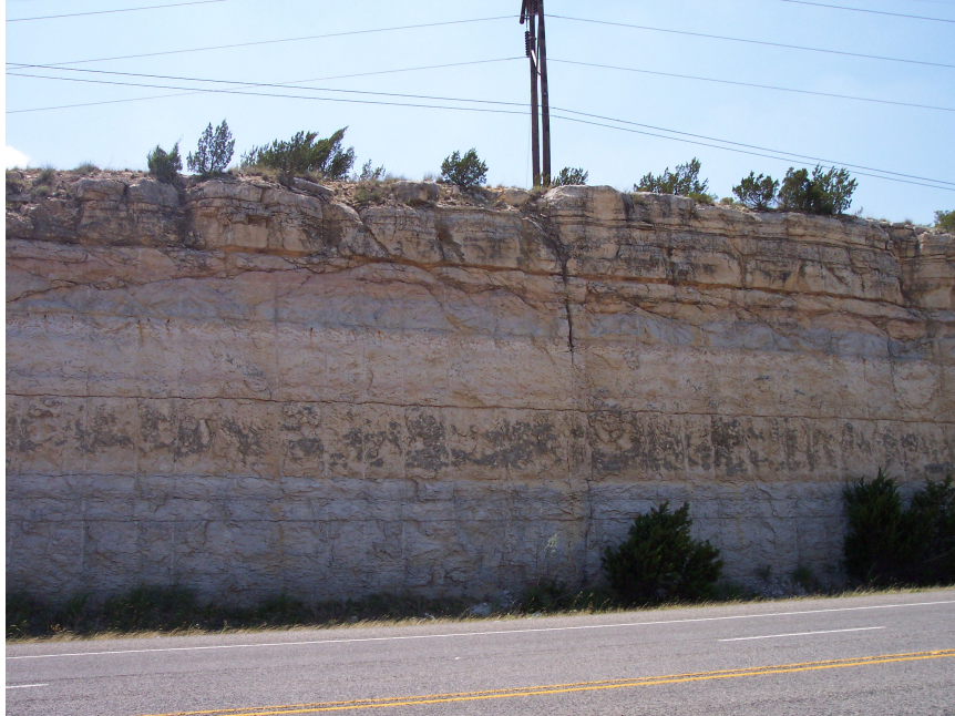
Figure 4.14. Photograph of feature in limestone showing obvious signs of large-scale water intake. Photograph taken by the author, US 277 in Schleicher County, Texas.
