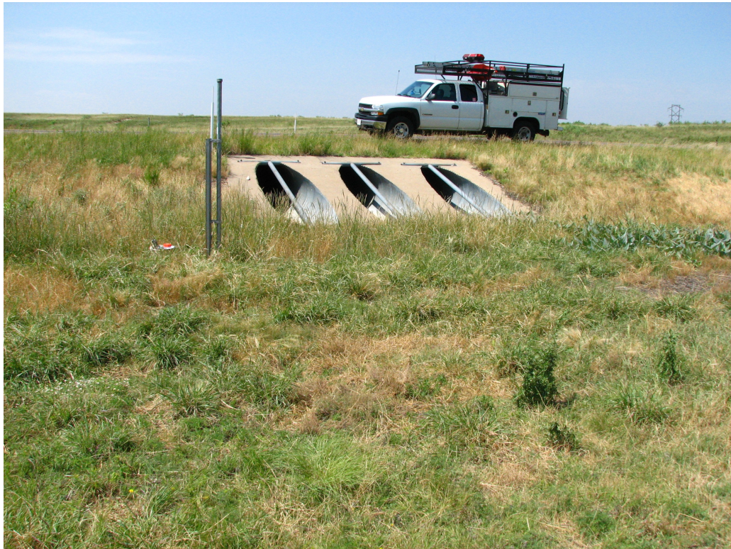
Figure 1.1. Photograph of U.S. Geological Survey Peak-Streamflow Station 08123618 Sulphur Springs Draw near Plains, Texas Courtesy of USGS Lubbock Field Office
