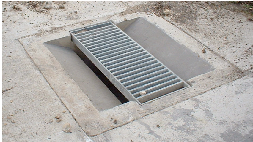
Figure 1: Type-H inlet located on I-35 feeder near San Marcos, Texas.
