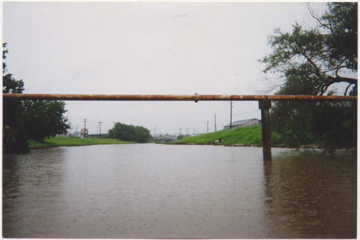
Figure 4: Column support used as reference for all water measurements at Station 1.
