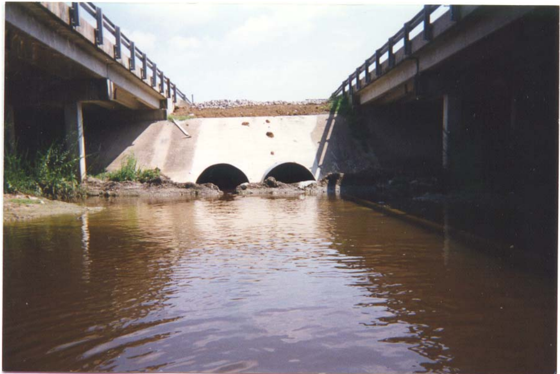
Figure 3: Drainage outfalls from the construction site as seen from Cow Bayou.
