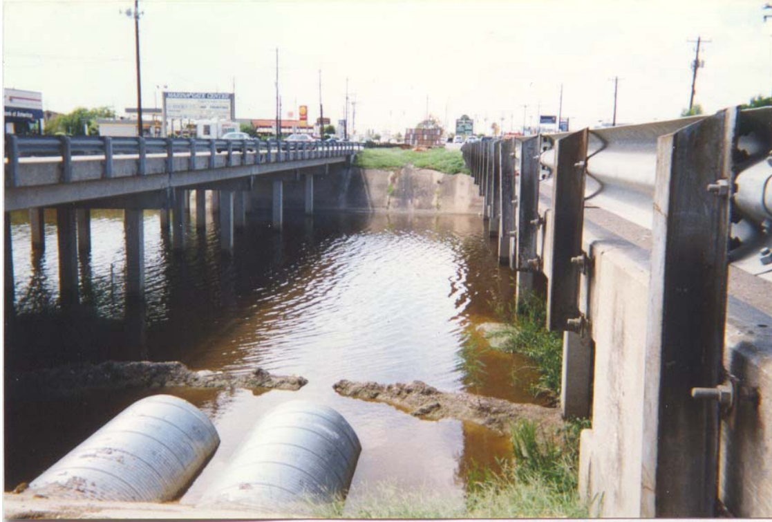
Figure 2: Drainage outfalls from the construction site as seen from NASA Road 1.
