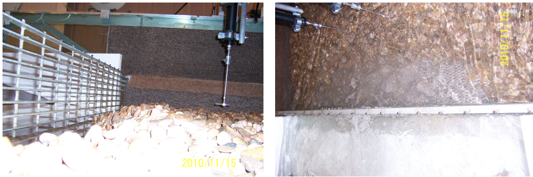
(a) Picture of the galvanized grate. (b) Water flow through the grate Figure 3.6. Dispersion grate
