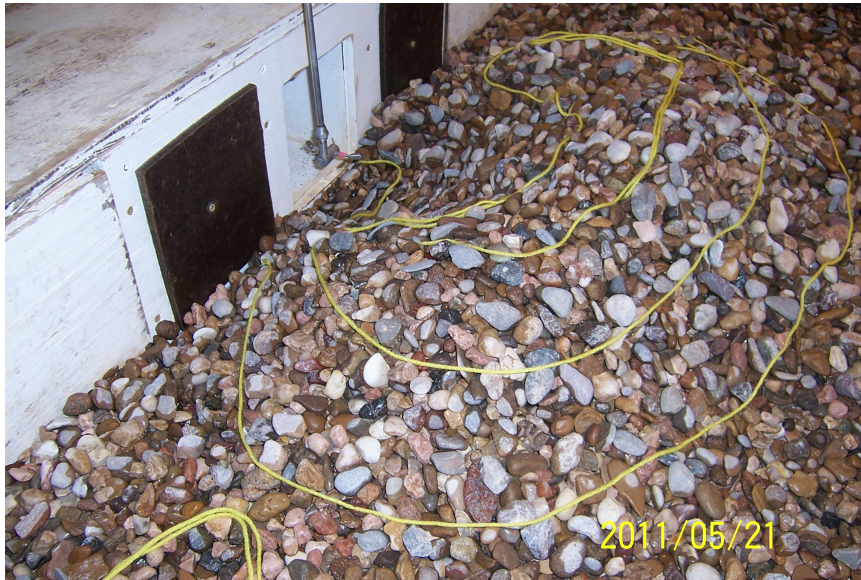
Figure 8.19. Example of the slope reversal on the downstream sediment dune
