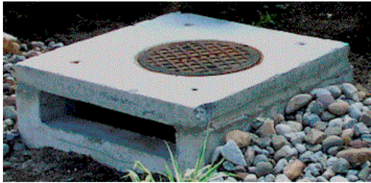
Figure 3. Grate-inlet (not Type-H) that is representative of the type of grate inlets that Type-H inlet (grate top) hydraulics is thought to mimic.
