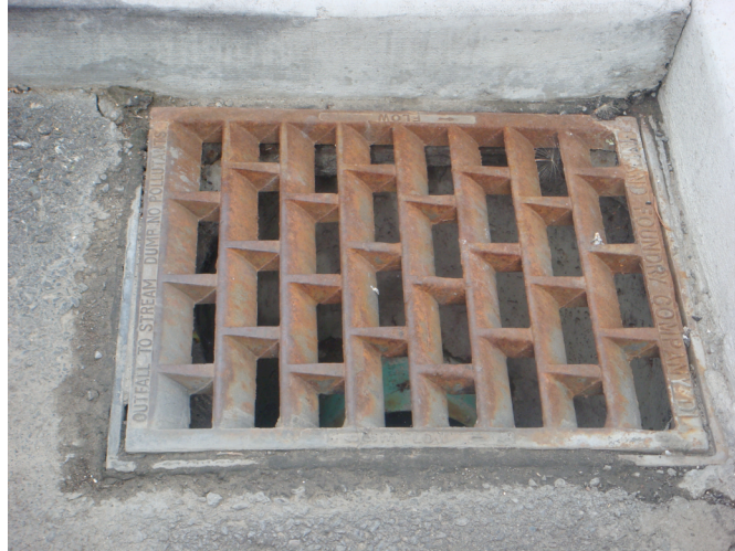
Figure 9. Slanted-vane type grate inlet.
