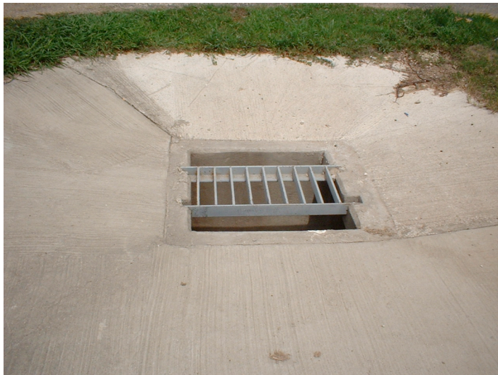
Figure 1. Representative Type-H Inlet (grate top) near I-35 at Jarrell, Texas.
