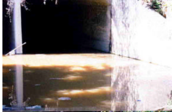
Country Club Bayou Outfall. Upstream of HB&T Railroad Bridge. March, 1998
