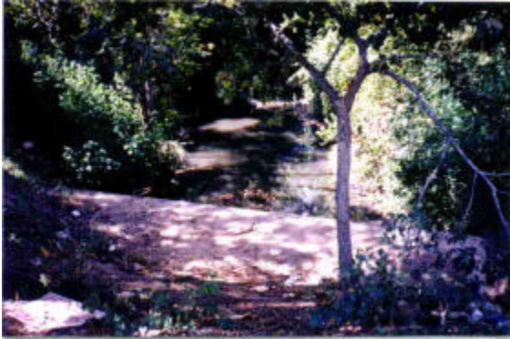
Looking upstream from culvert under Polk Street. March 1998
