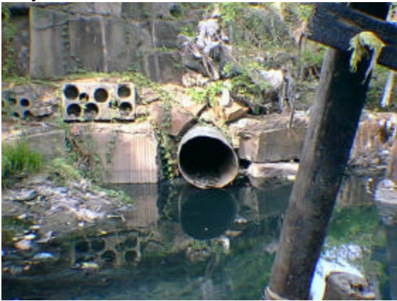
Culvert used to estimate water level for field notes May, 1998
