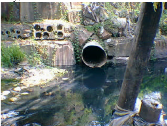
Culvert view May, 1998
