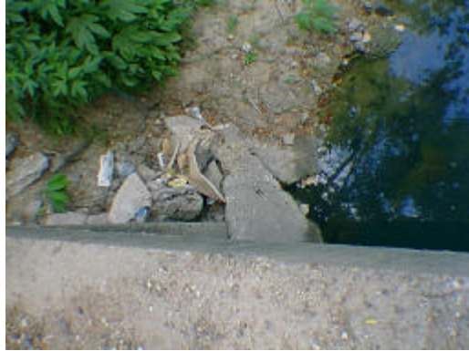
Looking down from culvert June, 1998
