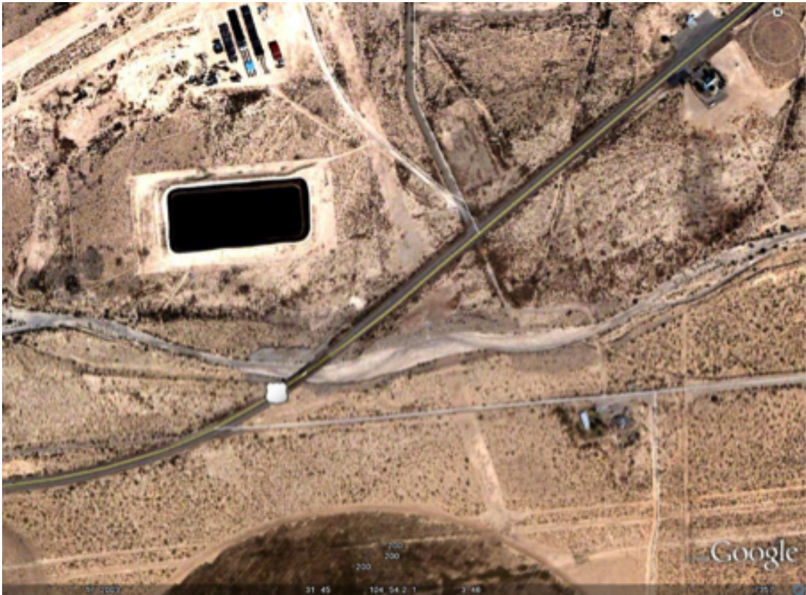
Figure 53: Google Earth aerial photograph of US 62/180 bridge over Guadalupe Arroyo, Culberson County, Texas
