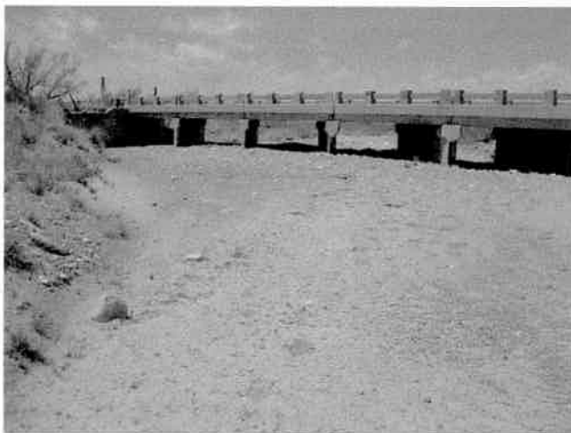
FIGURE 7 Guadalupe Arroyo at upstream crossing of SH-54, looking downstream (larger material in bridge vicinity; bankfull configuration is evident in stream adjacent to this bridge).
