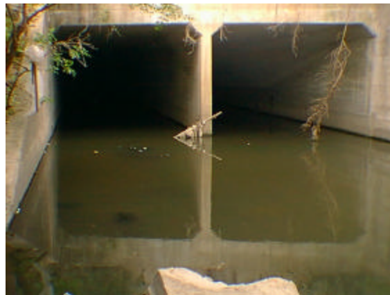
Figure 2. Hughes Street Outfall
